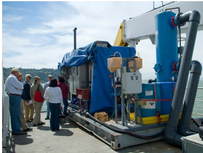
$1M retrofit allowing open deck installation of ballast water treatment systems
